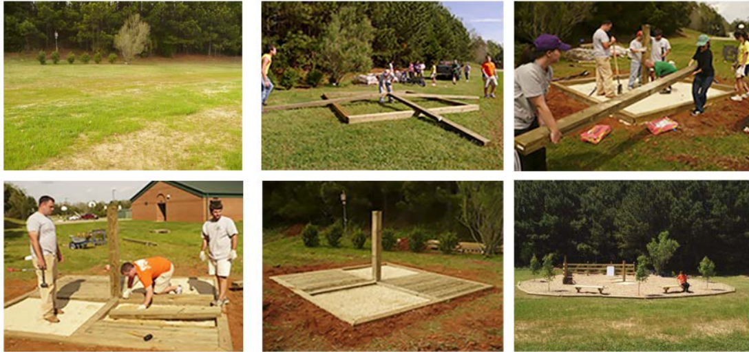
Figure 3.13 the LM garden constructing process
